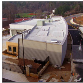
CDC Transshipping Facility
