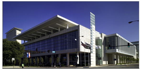
McCormick Place Convention Center- West Hall Expansion
